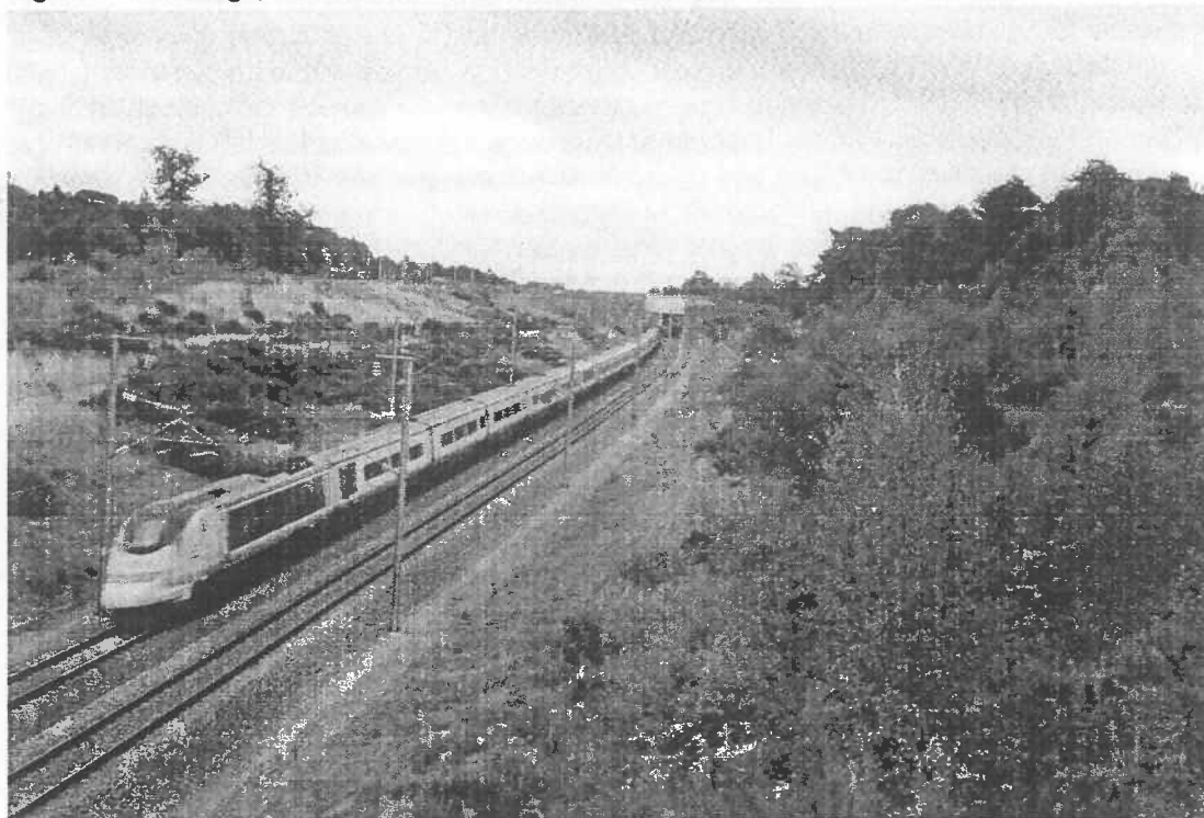
Figure 1 – Cuttings, like those used on HS1, would help to screen views [Arup]
